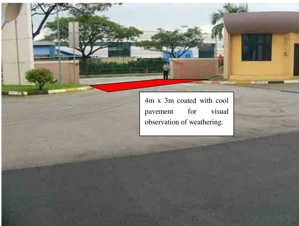
Figure 12. Driveway of Tuas road flatted factory.
